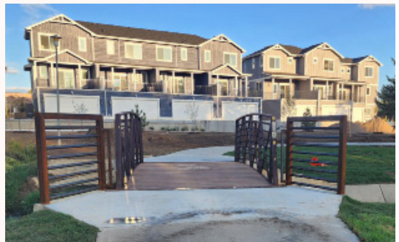
The Spangler Bridge, spanning Spring Gulch #1 in Northeast Longmont.
