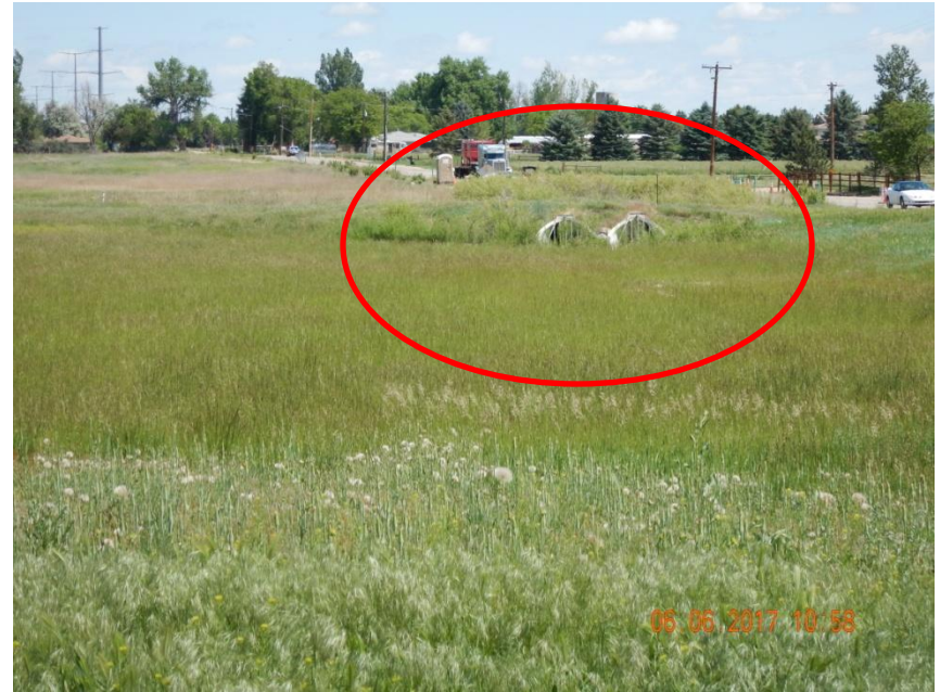
Photo 6. Photo taken of the access road entrance off CR 1. Culverts remain at location and have not been removed per Rule 1004.
