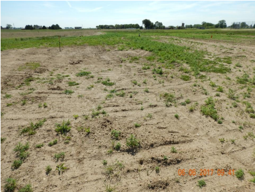
Photo 1. Photo taken from the northern well location, facing East. Does not appear final reclamation activities have been performed based on the lack of grass species and the abundance of weedy annuals, mostly Kochia.
