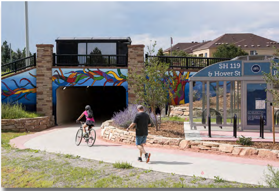
A new underpass on Hover Street adds safety for cyclists and pedestrians
