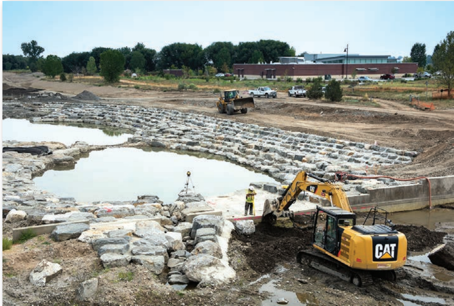
The Resilient St. Vrain Project includes creation of a new park and nature area.
