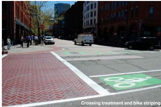
Crossing treatment and bike striping
