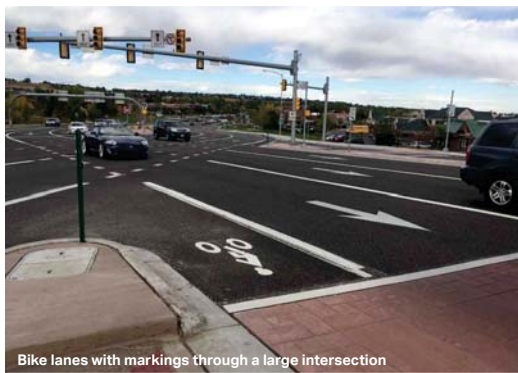
Bike lanes with markings through a large intersection
