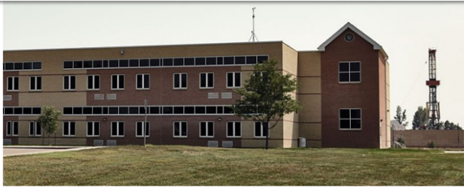
A drilling site operated by Extraction Oil and Gas sits just 1,300 feet from Bella Romero Academy in Weld County. / Anthony Camera
