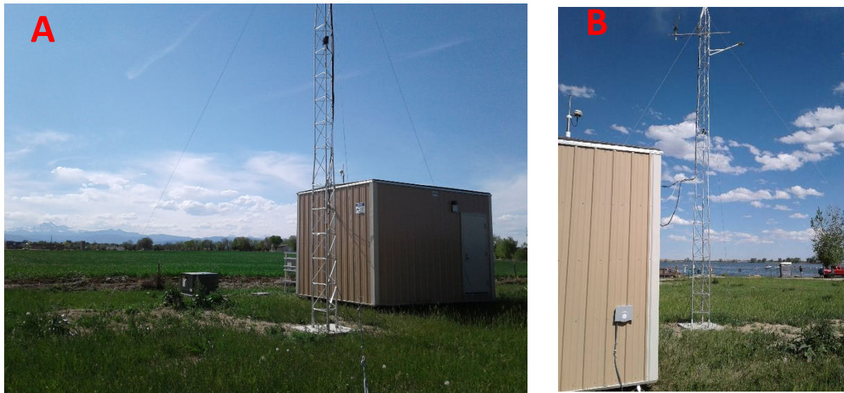
Figure 2: LUR Instrument shelter with adjacent meteorological tower looking towards the west (A) and east (B). The water surface of the Union Reservoir can be seen in the background of the latter figure.
