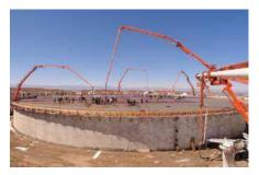
Figure 4-12: Construction of a Post-tensioned concrete tank
