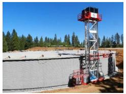
Figure 4-8: Type 1 winding machine
