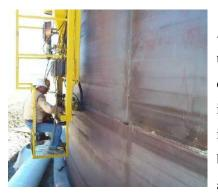
Figure 4-2: Automated Welding for a Steel Tank Shell
