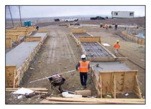
Figure 4-10: Layered precast wall casting beds
