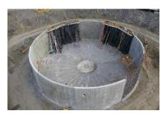
Figure 4-6: Cast in Place Conventionally Reinforced Concrete
