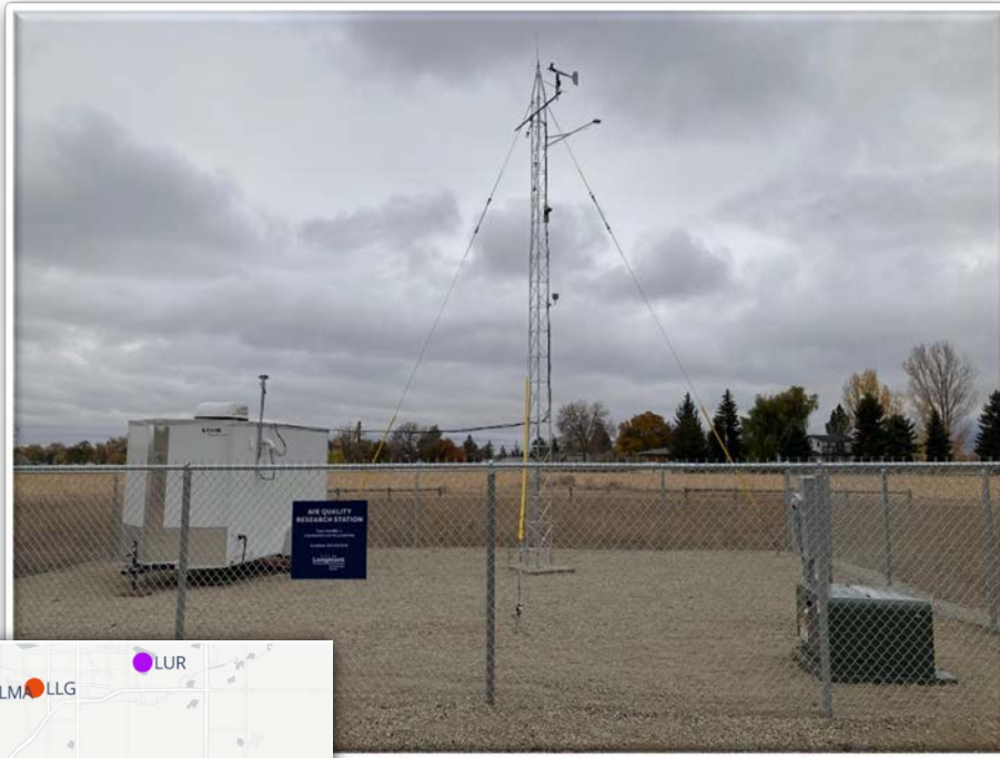
LLG after installation (photo by Jacques Hueber)
