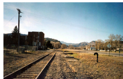
Railroad corridor adjacent to Highway 66 (recommended route F-1).
