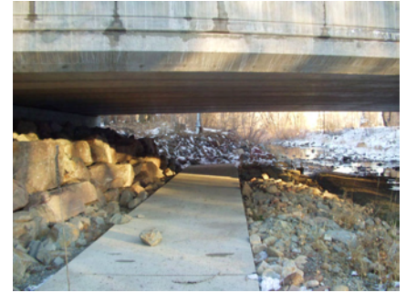
Existing underpass at US 36.
