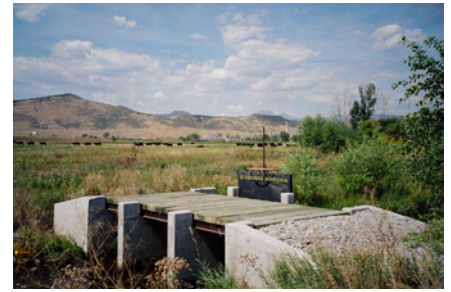
Existing bridge over the James Ditch (Alignment E-7).
