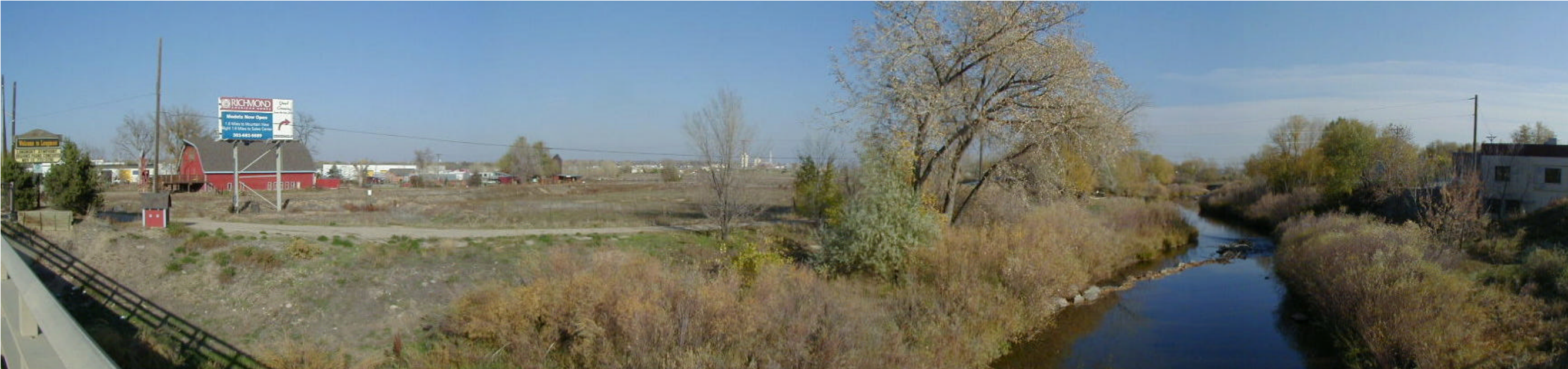
Panorama looking east from Main Street bridge located within the Urban Reach
