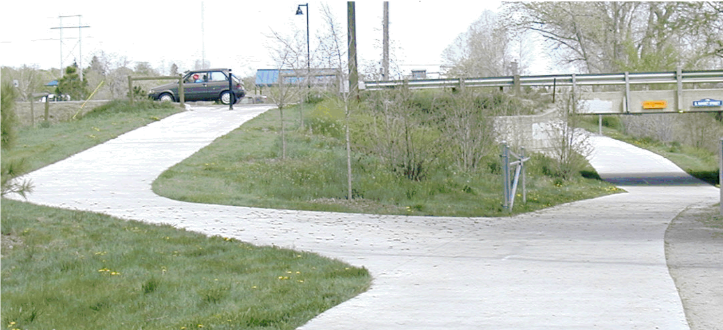
Existing ramp along the built portion of the Greenway
