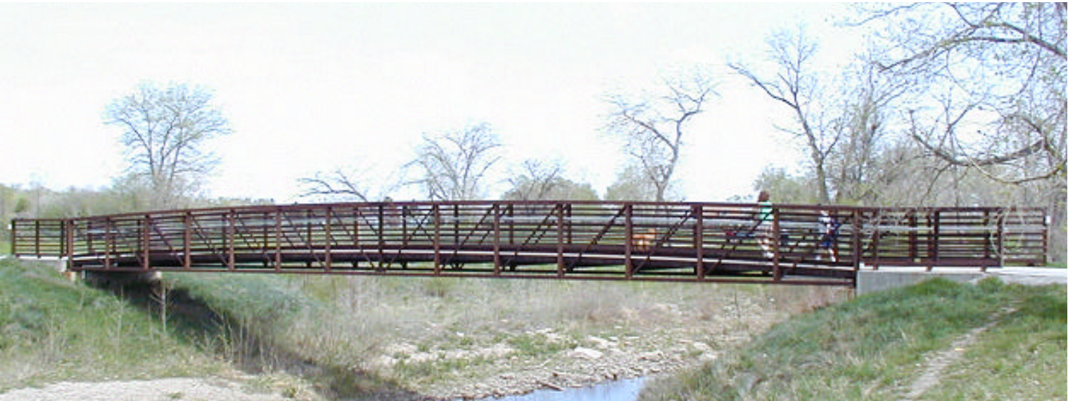
Pedestrian Bridge - the free span, Cor-ten steel bridge with wood decking is available from a variety of manufacturers including Continental and Steadfast.
