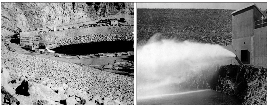
Figure 58. (Left): Button Rock Dam stilling basin and outlet works (1969); (Right): Outlet works bypass pipe, used during low water demand periods. The square opening, designed for a greater volume of water, is used during high water demand periods (1974) (Longmont Museum & Longmont Times-Call collection).
