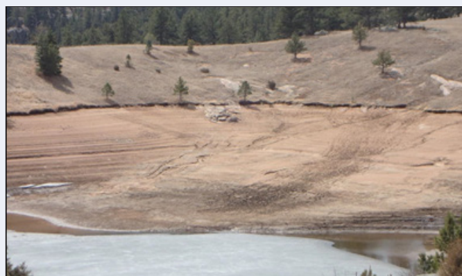
Figure 43. View of rilling through reservoir sediments from overland flow (Photo SB01, RiverRestoration, 2019).
