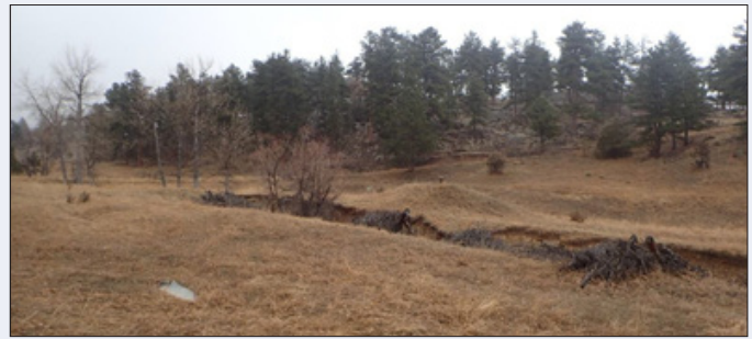
Figure 39. Head cutting and placed wood piles as an erosion control measure (Photo NB14, RiverRestoration, 2019).
