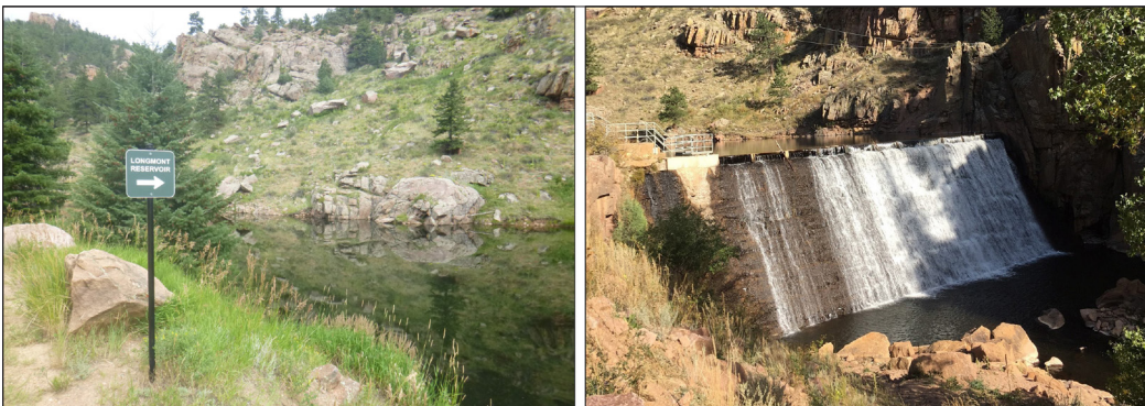
Figure 63. Longmont Reservoir and Dam.
