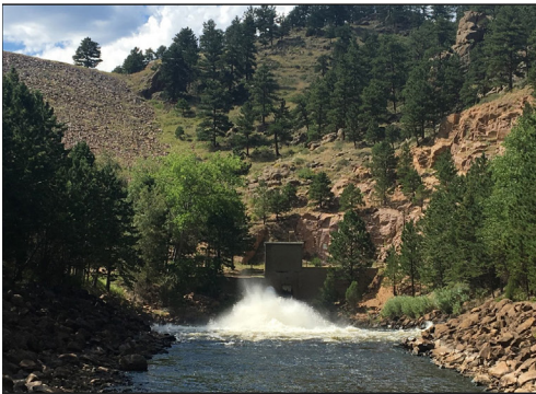
Figure 60. Exterior and interior views of the reservoir outlet house at the base of Button Rock Dam.
