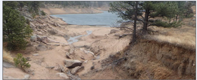
Figure 40. Channel form and avulsion at stream outlet into Ralph Price Reservoir (Photo NB05, RiverRestoration, 2019).
