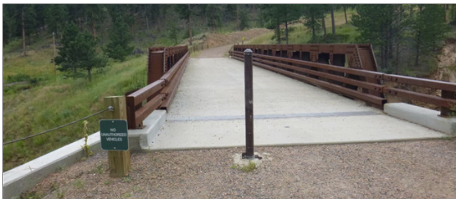
Figure 76. Looking south at the spillway bridge and removable bollard.
