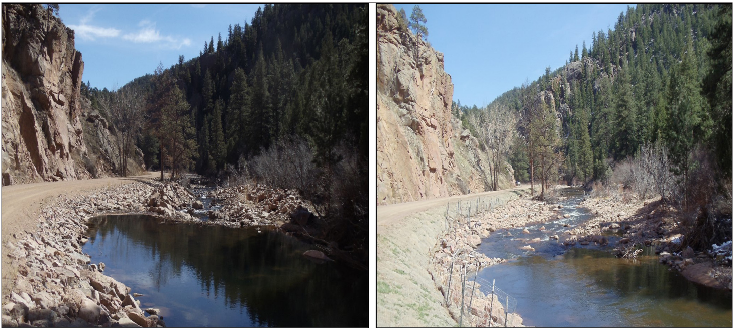
Figure 70. Phase 1 restoration before and after, looking downstream. The left photo (March, 2016) shows the overly wide channel planform and a riprap slope with no vegetation. The right photo (March 2017) is one year later. Sediment deposition had been removed from the channel, the left bank is seeded with erosion control measures in place and native riparian shrubs are planted on both banks.
