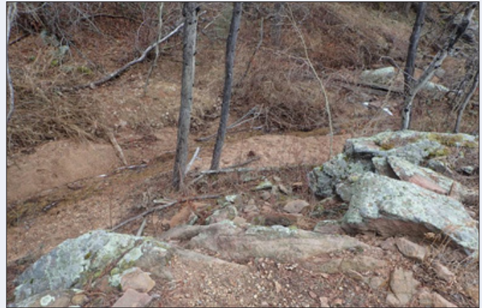
Figure 31. Sand and gravel deposits in channel from adjacent road/trail (Photo CT6, RiverRestoration, 2019).
