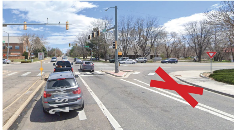
Removal of Channelized Right-Turn Lanes
